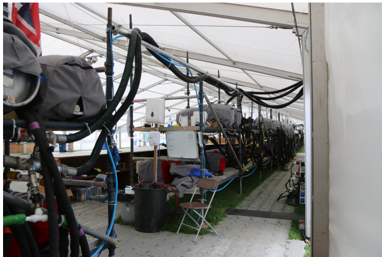
Pipes entering the marquee and crossing the stillage gap on a 6 m tube
