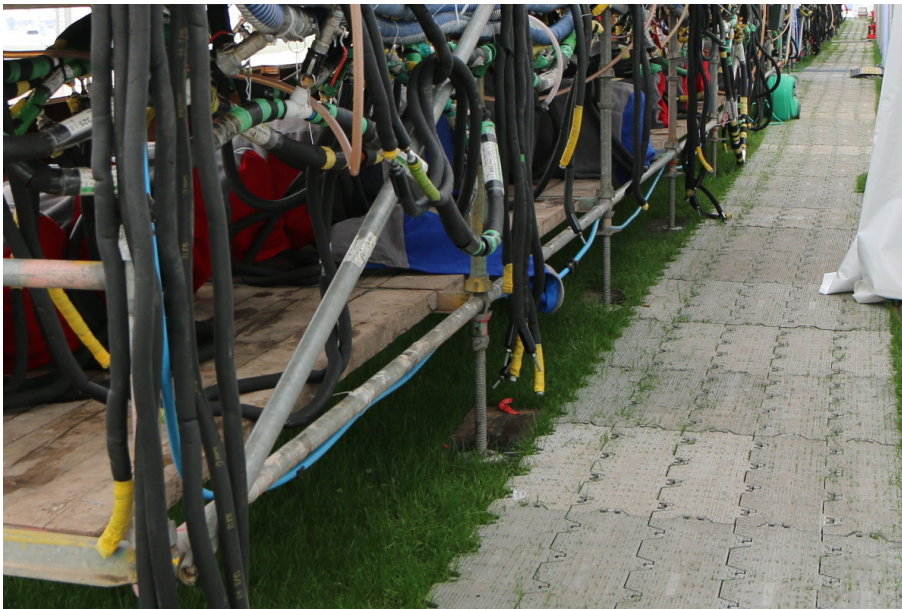
Pipe regularly secured to ledger, raised from ground contaminants
