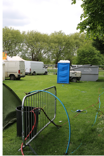
Tap raised and secured away from contamination, pipes and cables away from vehicle crush risk and (most) people's feet
