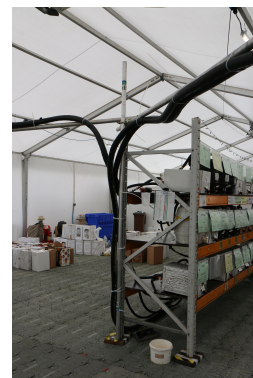
Vertical scaff. pole used to reach Cider
