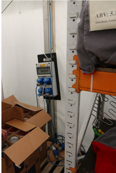
Distribution board upright near stillage, remaining accessible and free of a beery-bath
