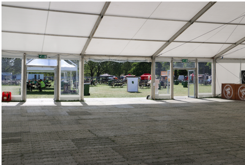
Emergency exit signs suspended over and wired along the inside eave-rails, over the roll-up wall
