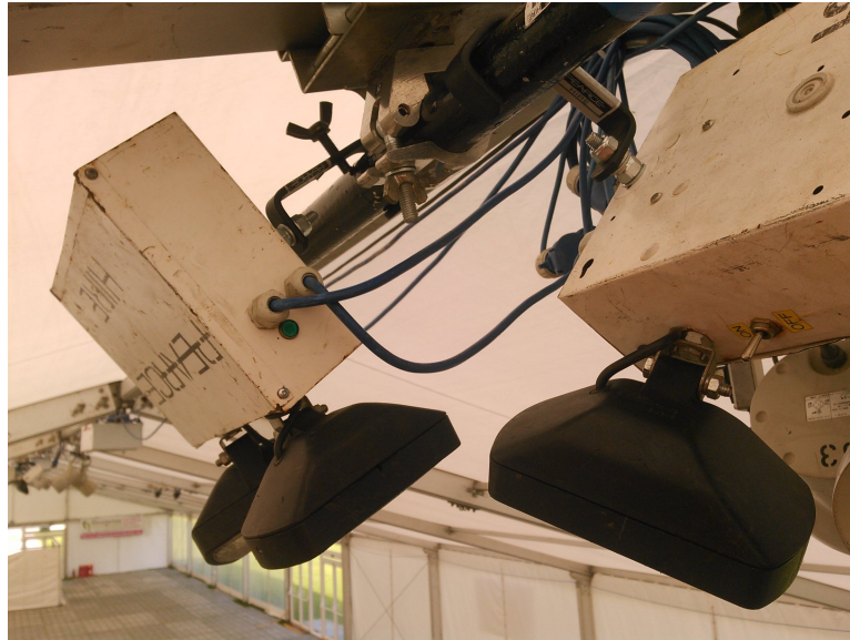
Two twin-head units mounted using a keder clamp
