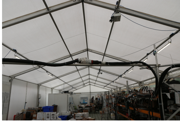
Cider and foreign bar lighting. Note the twin-head units.
