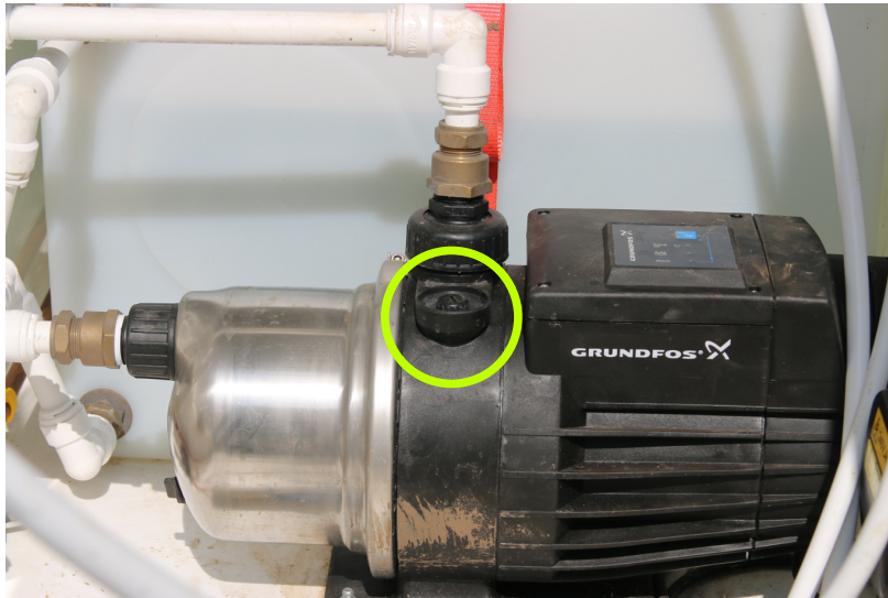
Shower pump, priming plug circled
