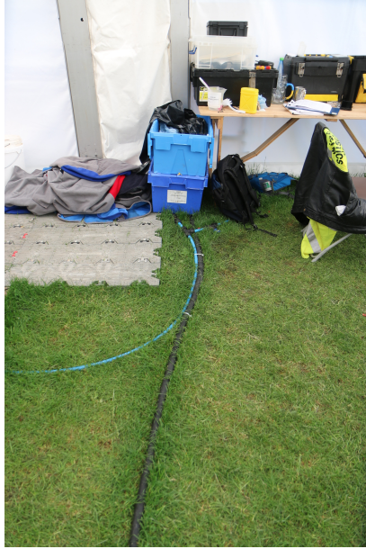
Springy water pipe tied to heavy cable, reducing trip hazard
